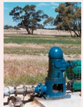
A CF75 fitted to a 150mm line.
