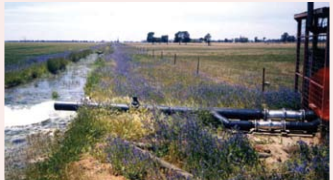
A CF150 and CF100 were manifold together to deliver 4,400 and 2,200 lit/min respectively (9.5meg/day). Headloss 27kPa – no orifice.
